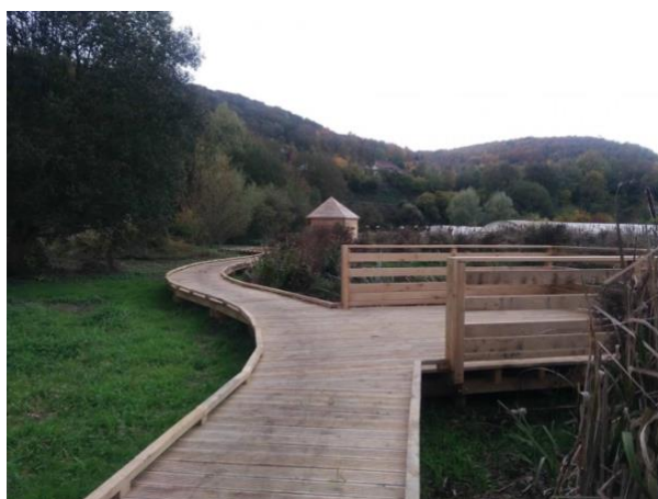
Box 1: Wetland of Repainville (Rouen, France)
